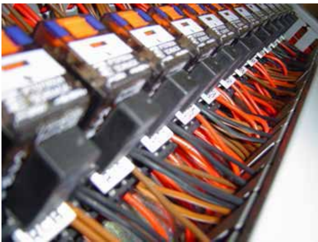
detail of connections in the old control board
